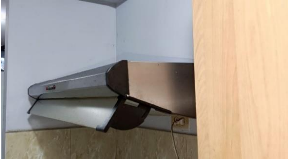
Figure 5. Sample of ductless range hood used in Panama.
